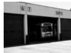
Sample Transit Facility.
